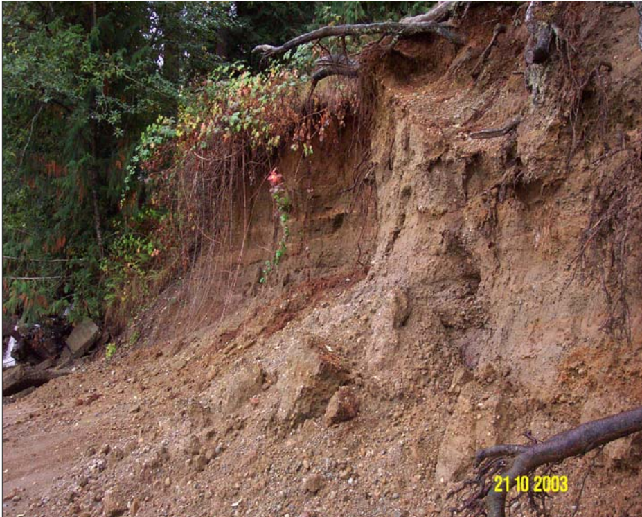
The picture illustrated below shows bank erosion at Walker Park
