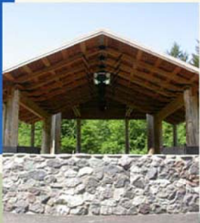
Environmental Learning Shelter-Orientation Kiosk under canopy
